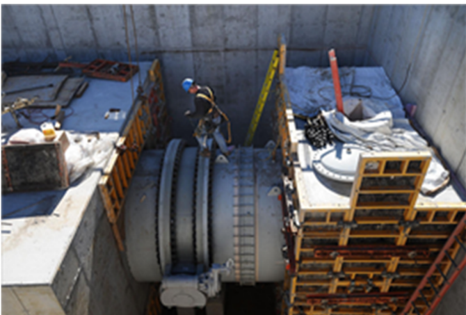
MWWST Valve Vault and Pipeline
